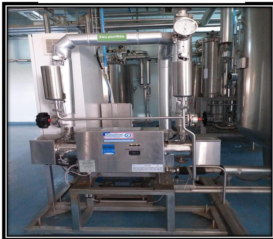
Figure 22 : Machine ultraviolet
